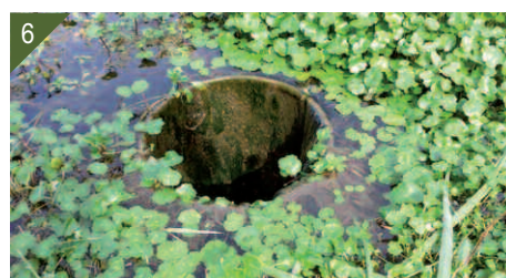
5. Cutting of water pennywort. 6. Overflow outlet of the Lagrollet Pond invaded by water pennywort prior to the installation of screens.
